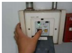
Figure 9. Function test manual pull station
