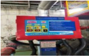
Figure 25. Control panel for engine pump & jockey pump must be upgraded
