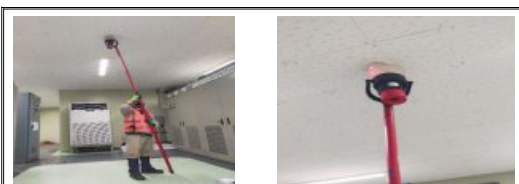
Figure 1. Function test smoke detector
