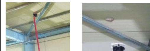
Figure 3. Function test heat detector
